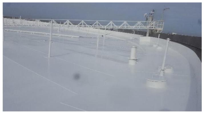
Floated roof appearance after polyurethane top paint
