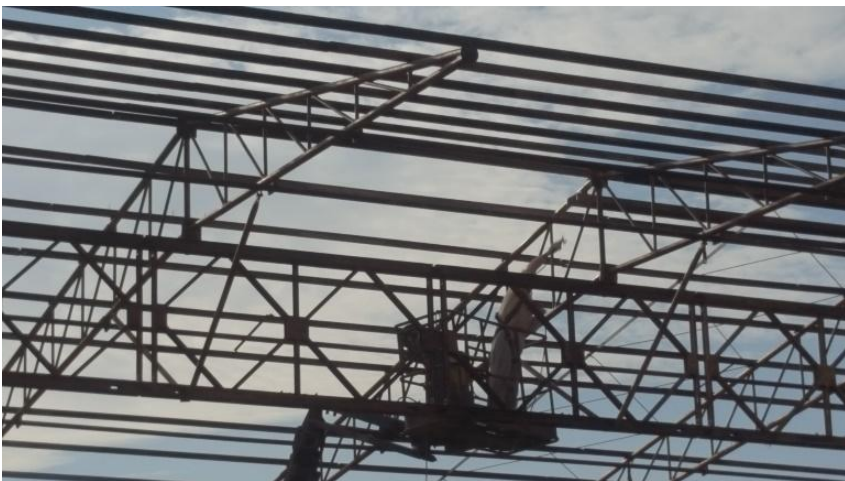
Single layer application with Airless
